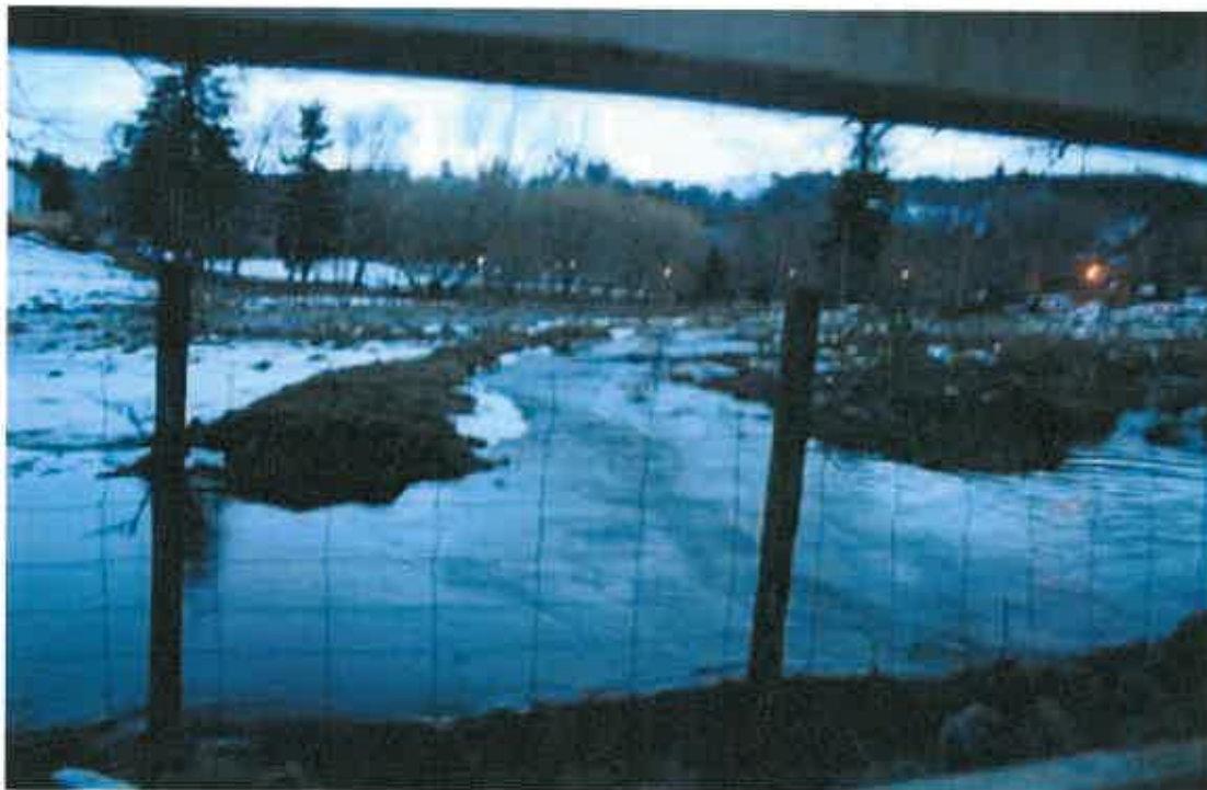
View from the bridge on The Dulaig's driveway, looking up the burn to Revoan. Note the significant flooding to the right (north side) of the burn.
