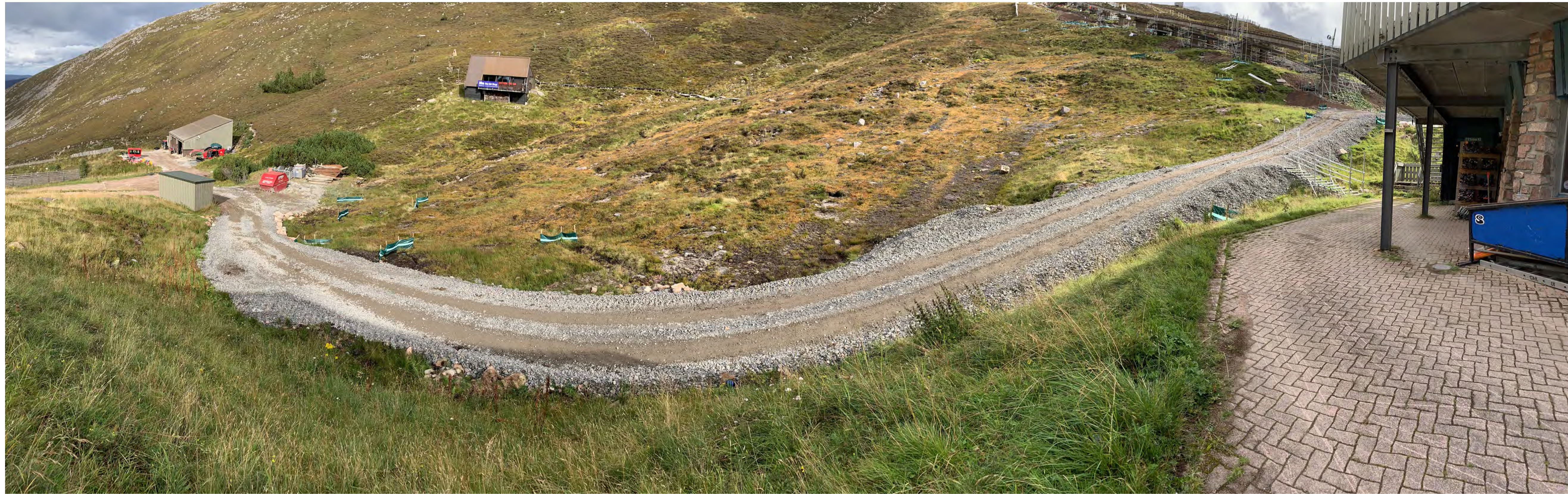
Existing temporary track view
