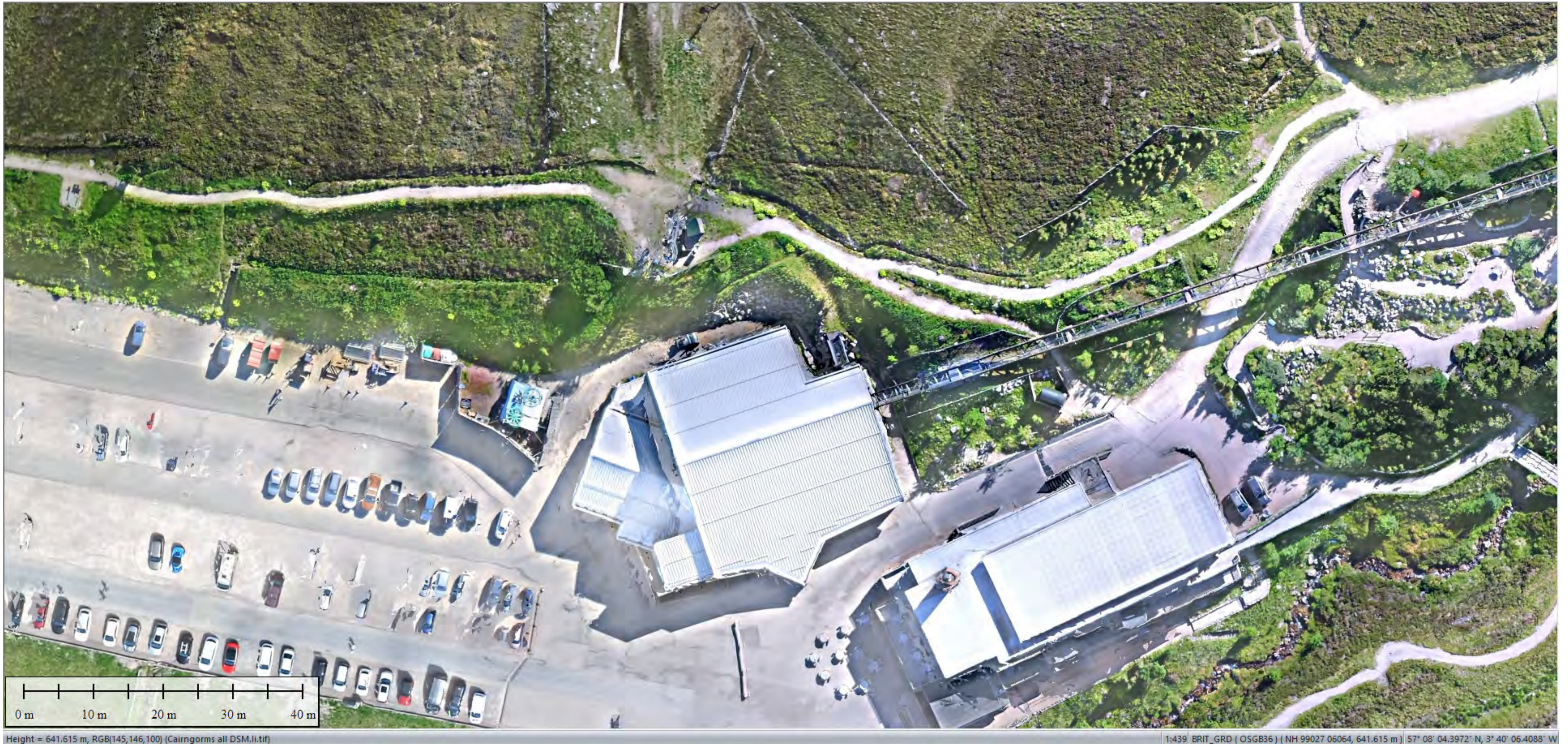
Existing aerial view
