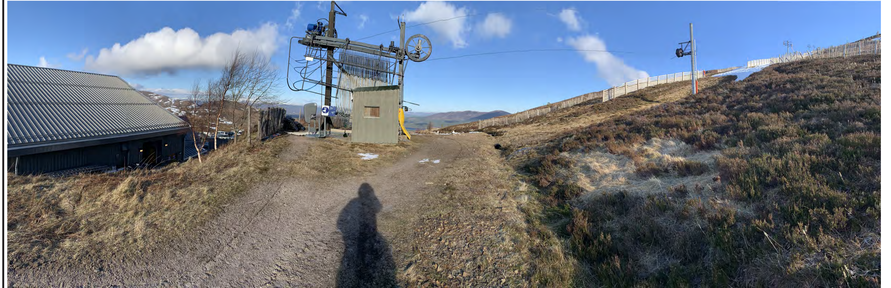
Existing View North East
