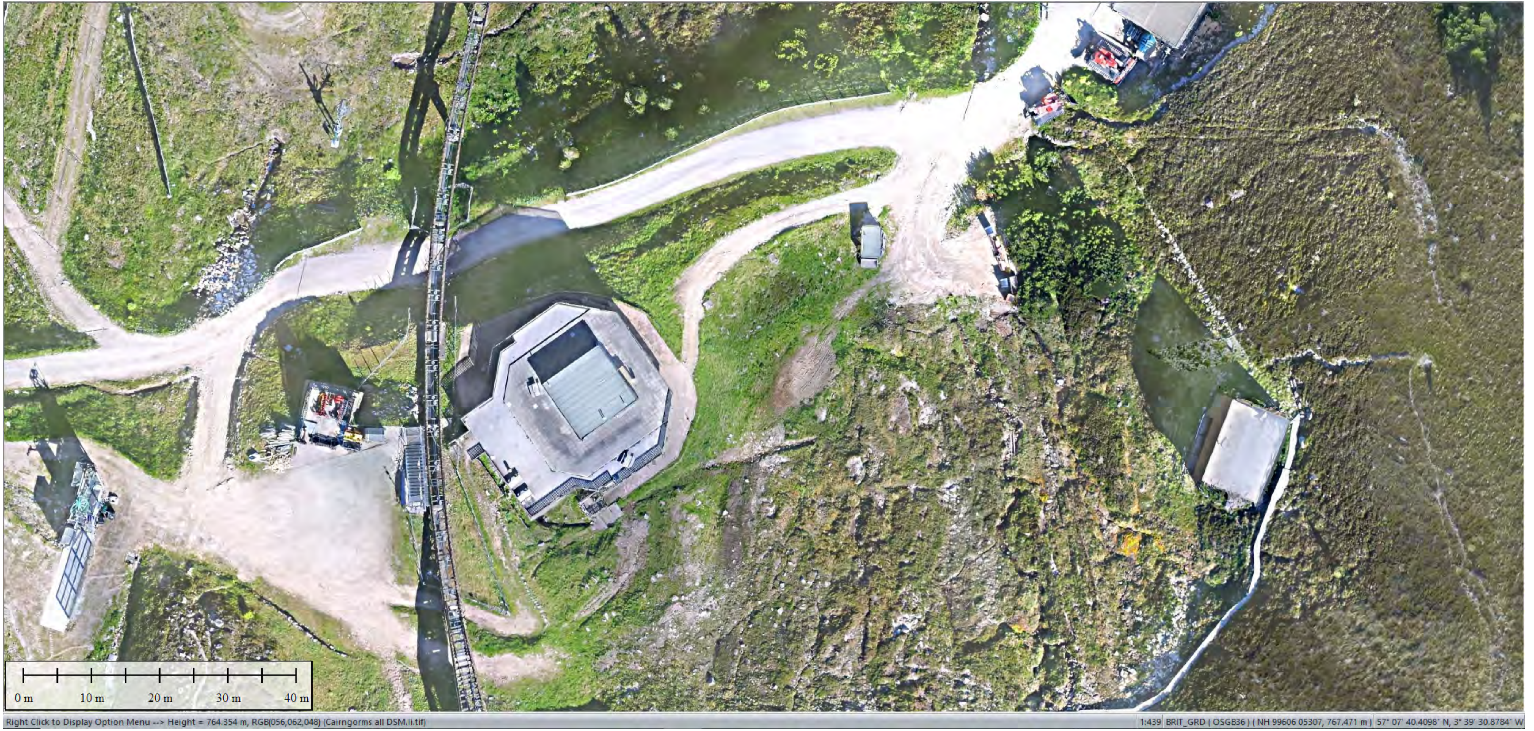
Existing aerial view
