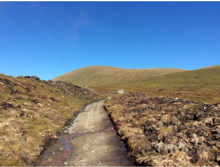
2 example photos of the above track specification
