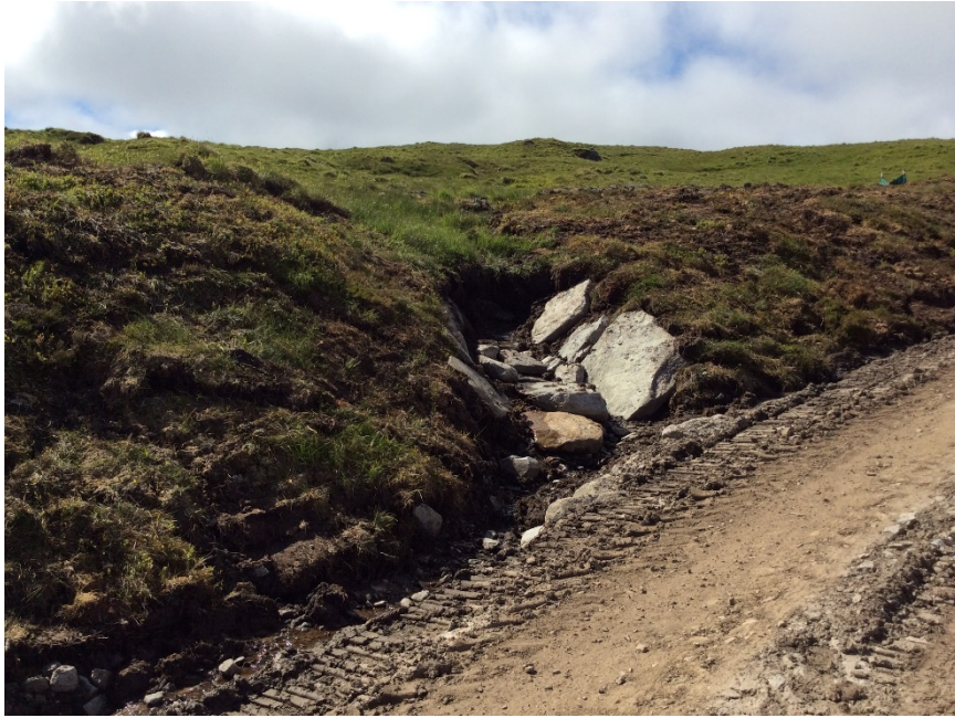
Example 1 of re-vegetating works using turves.
