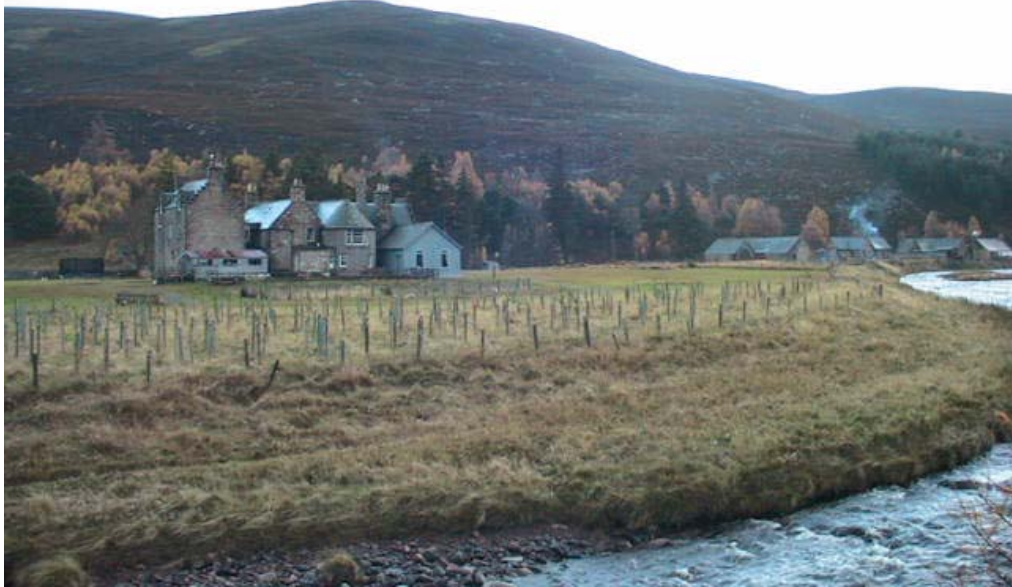
Fig. 3. Gairnshiel Lodge and adjacent buildings from the north
