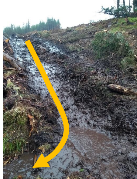
Forwarder Tracks Can Easily Become Pathways for Silt and Mud
