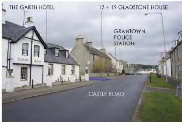
01 - VIEW FROM CASTLE ROAD TO GARTH HOTEL + GLADSTONE HOUSE
