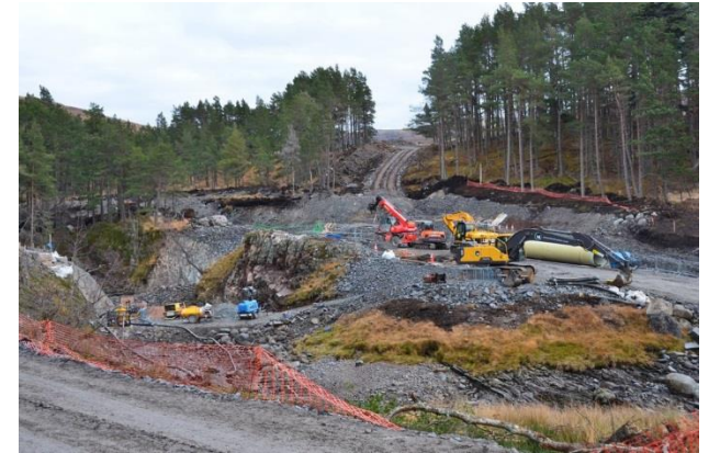
Figure 2 –hydro-electricity construction site
