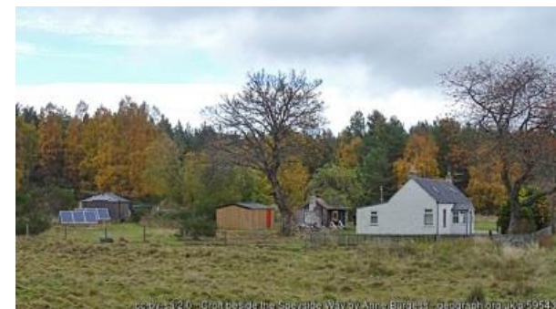
Figure 6 – example of ground mounted domestic solar panels (far left)
