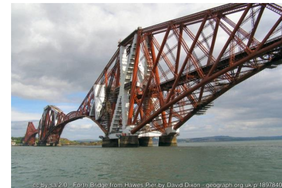
Figure 3 – perhaps the most infamous repair project in Scotland, painting the B listed Forth rail bridge (now done on a ~20 yearly basis)
