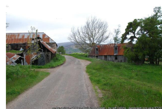
Figure 12 – BARR listed derelict farm at Upper Tullochgrue, near Aviemore
