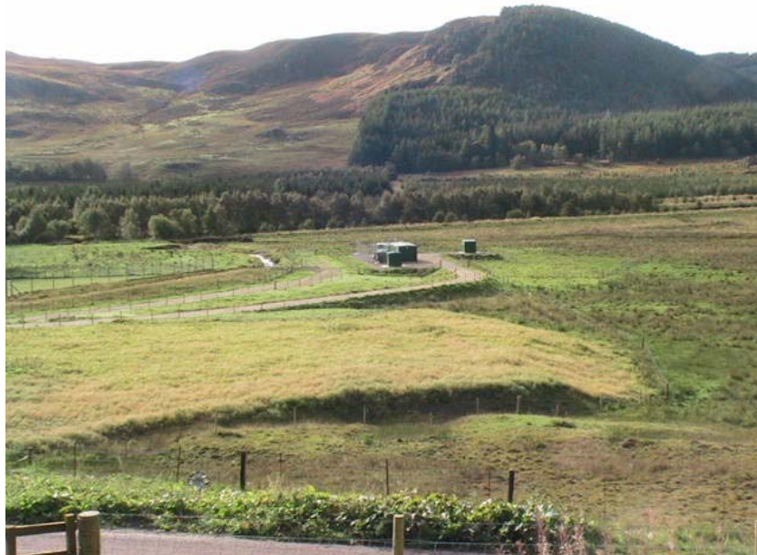
Fig. 5. Deposited Excess Material in Foreground
