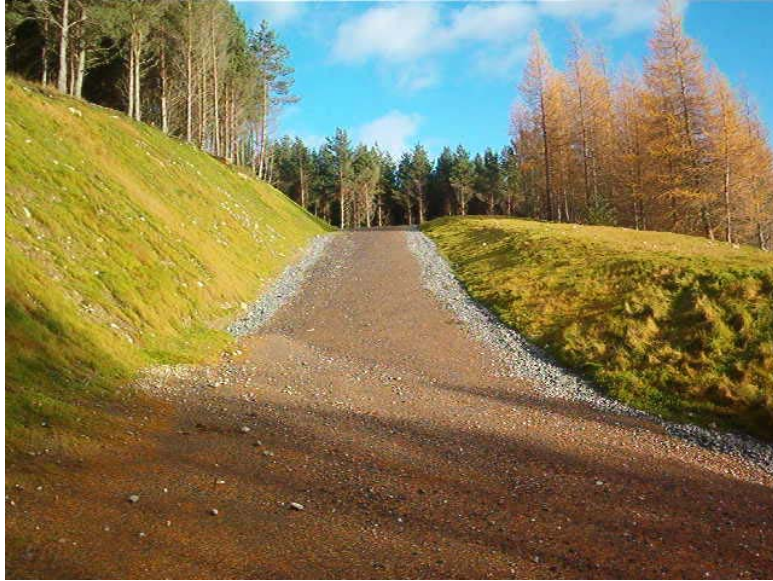
Fig. 7. Access track and cuttings
