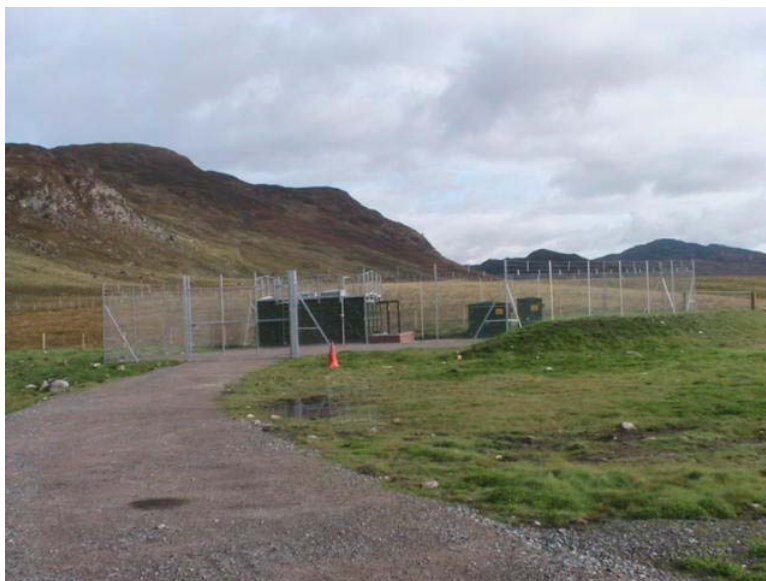
Fig. 4. Clear Water Tank Compound Looking East
