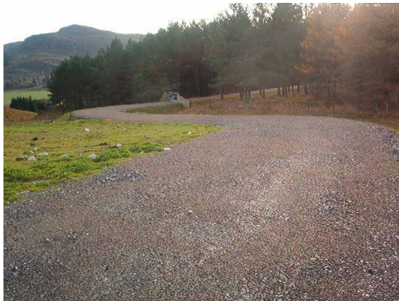
Fig. 10. Access track on approach to clear water tank compound
