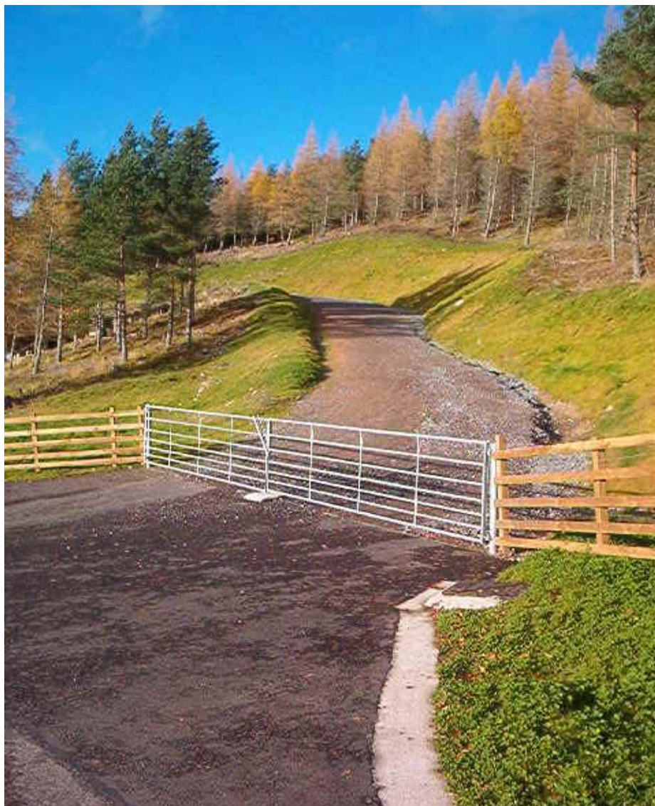
Fig. 6. Access track adjoining the public road
