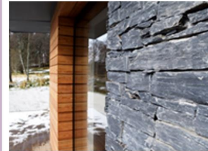
Stone and Timber on Contemporary Design, Strathdon
