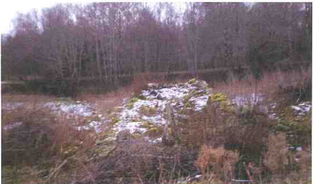
Figure 5 - Existing Site view illustrating ruins of Meall Mill
