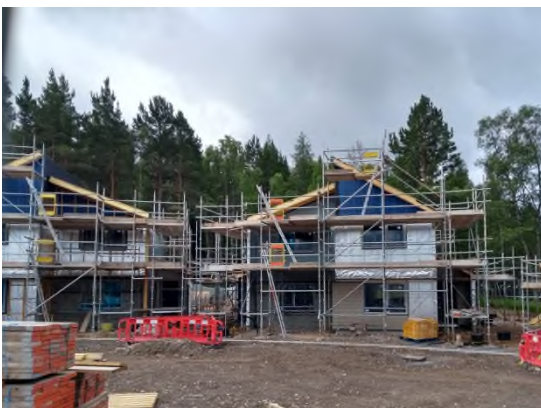
Figure 2 – affordable housing under construction at Inverdrue, near Aviemore
