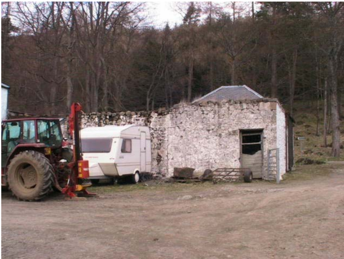
Fig. 4 - View of Courtyard elevation of building
