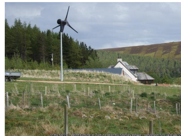
Figure 4 – free standing small scale turbine
