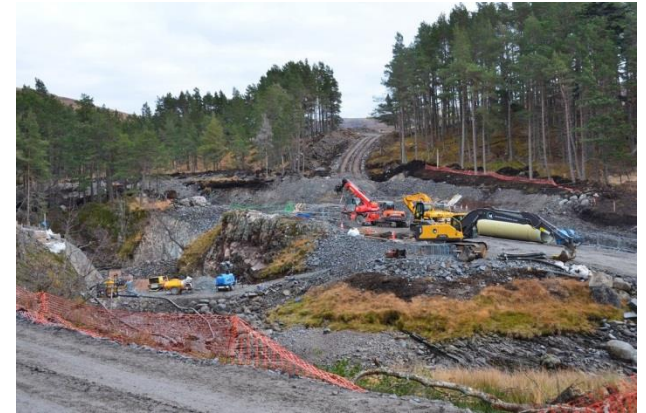
Figure 2 –hydro-electricity construction site
