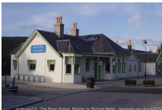
Figure 4 – Ballater old station, partially repaired, re-purposed and replaced after fire
