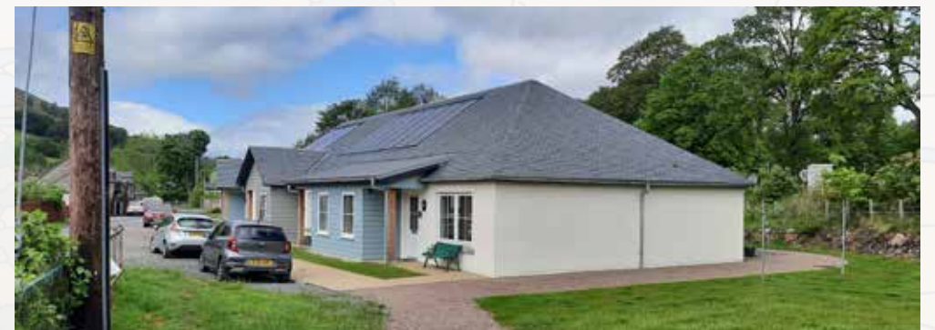
Images: Completed H3 Site, May 2022
