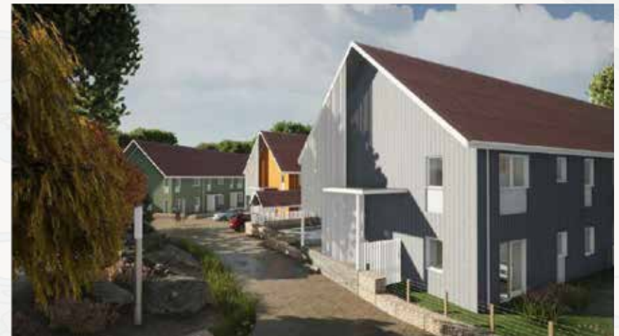
Above images from the Design and Access Statement submitted with application 2021/0166/DET
