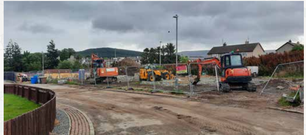
Site H2: Ground works underway on two further plots, August 2022
