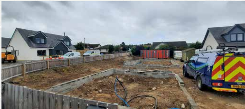
Site H2: Work underway on new plot, August 2022
