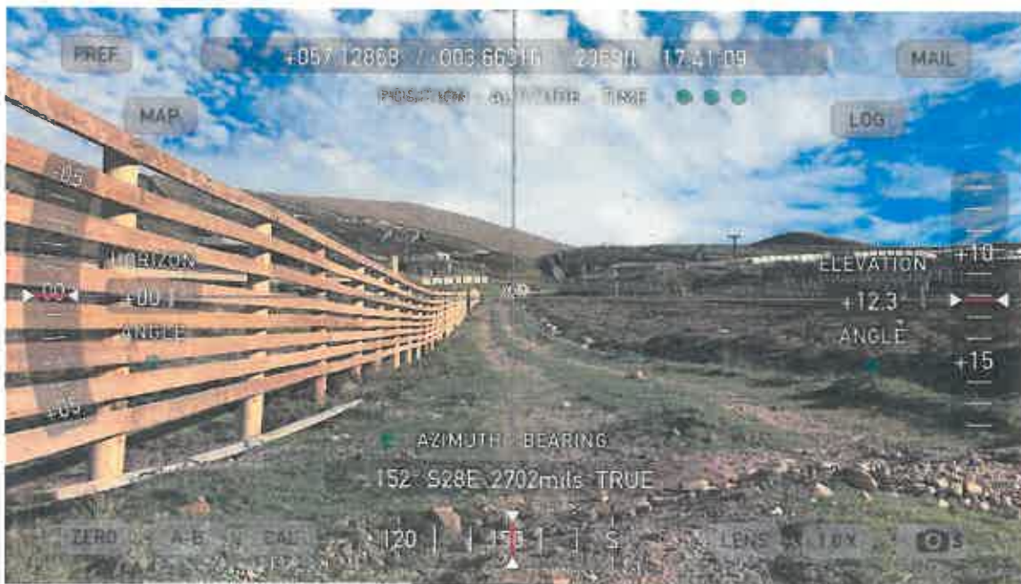
Image 4: Top half of the Sheiling Track averages a gradient of 12° exceeding that recommended as the limit in the SNH good practice guide "Constructed tracks in the Scottish Uplands" by 50%.
