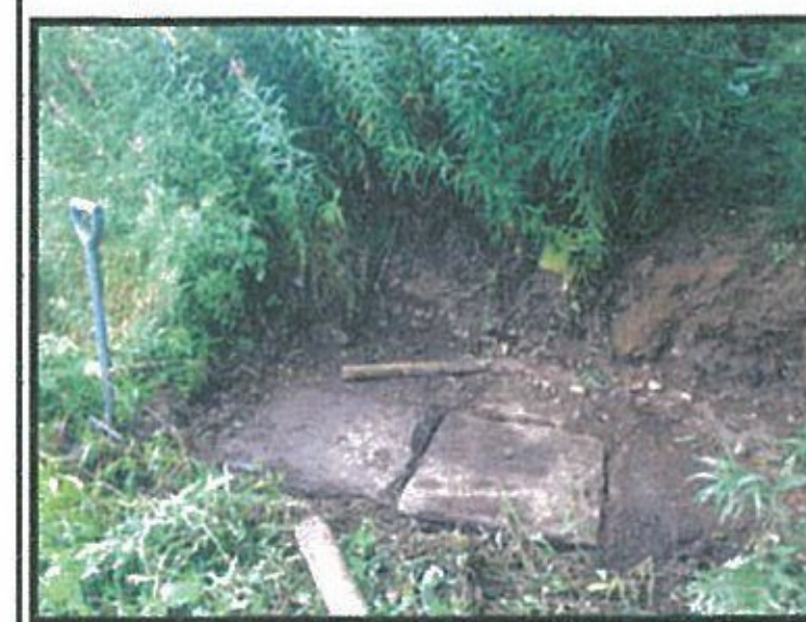
Original stone built septic tank
