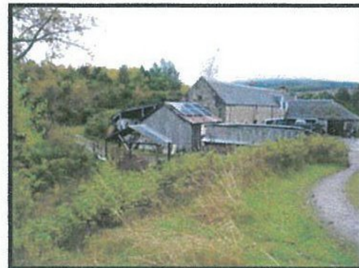
View of the back of the Garage
