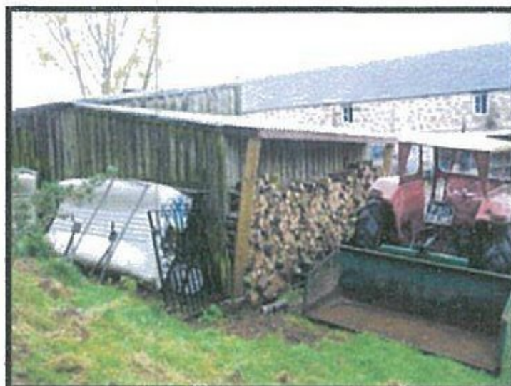
Existing Wood shed
