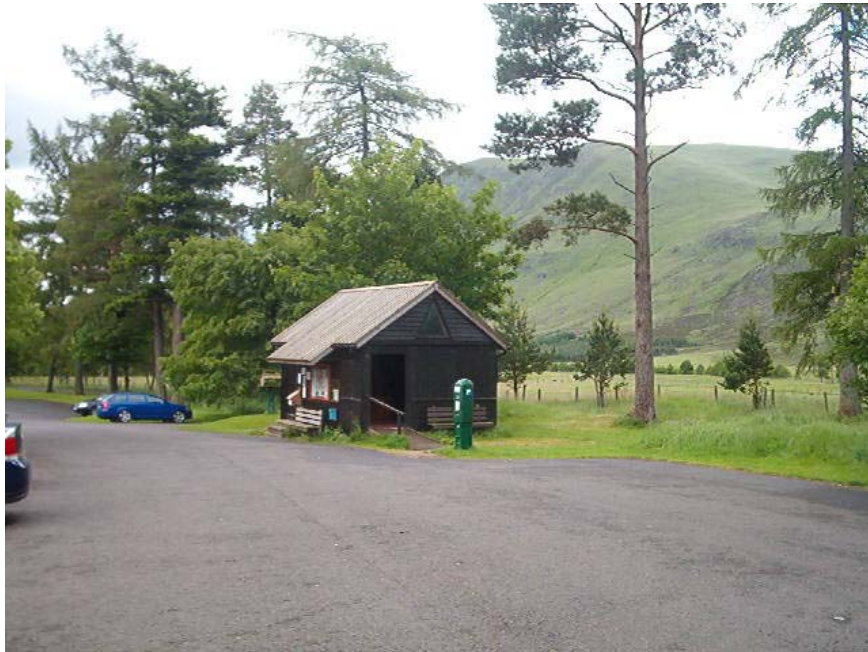
Fig 3 Existing information building
