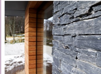
Stone and Timber on Contemporary Design, Strathdon
