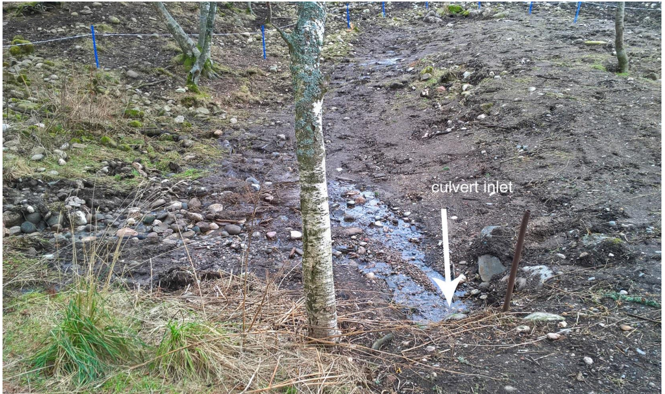
Figure 2: Photograph of culvert inlet within application site
