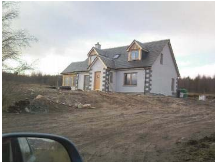
Fig 3 House substantially completed Feb 2010
