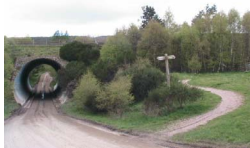
Fig. 5 : Milton Underpass providing access to the area at present.
