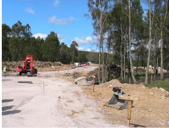
Fig. 3 : Southern area of the site – access road serving plots 46 – 75.
