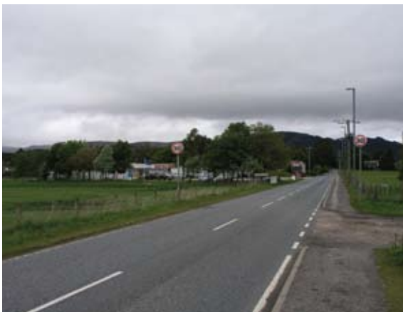
B9150 Perth Road link road access to left
