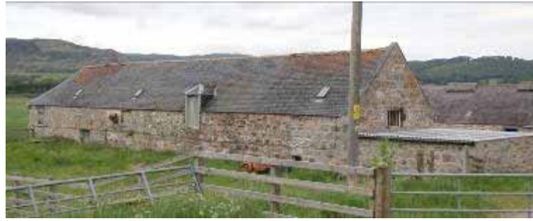
Fig. 6 : existing south west elevation (external view)
