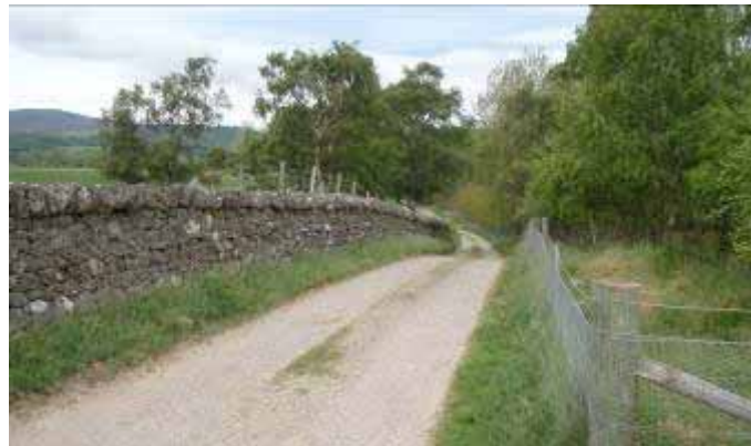
Fig.12 : Existing access track
