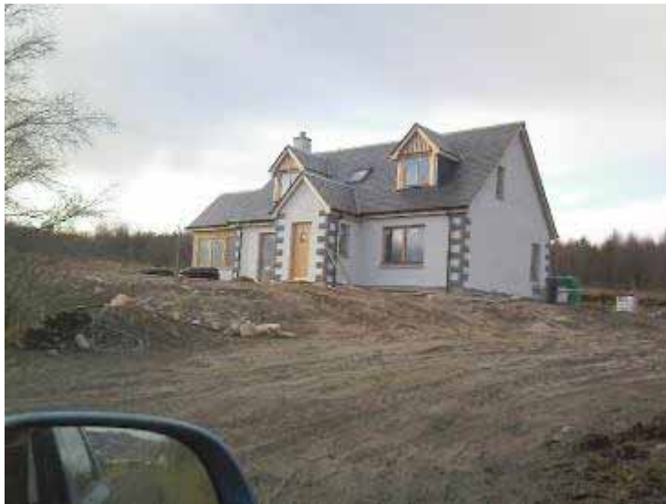
Fig 3 House substantially completed Feb 2010
