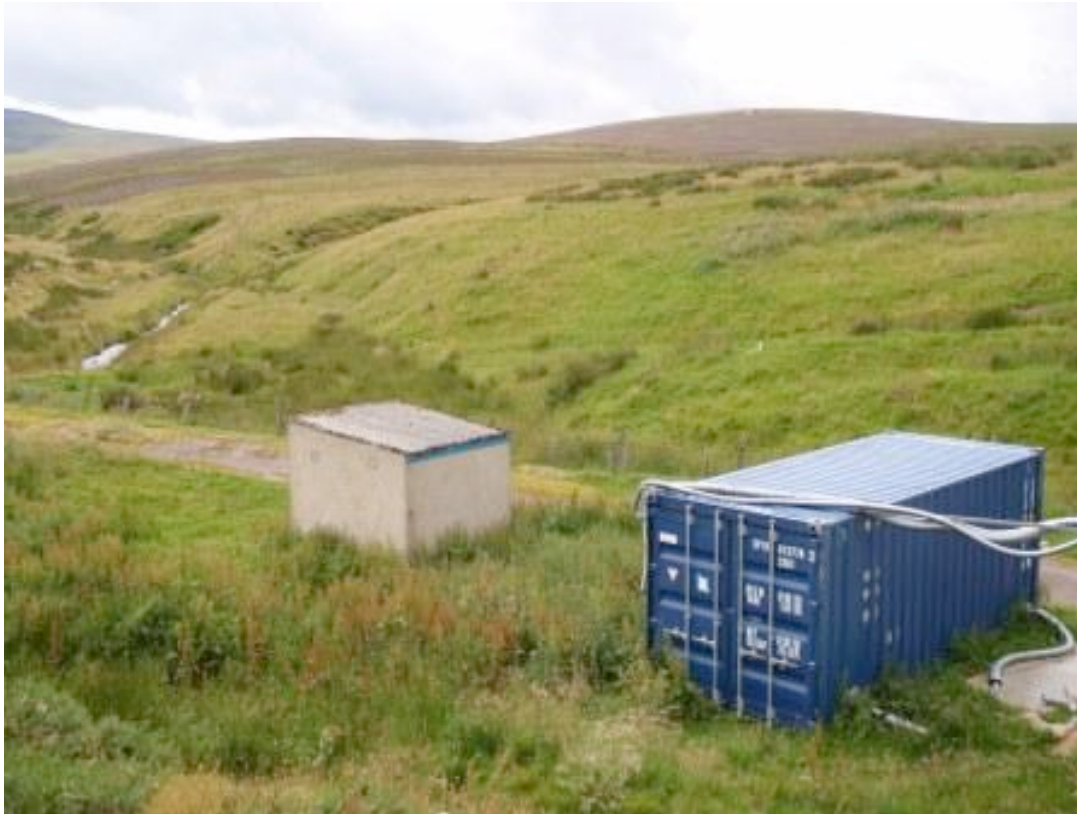
Fig 4 Existing water treatment buildings to be removed and location of new Water Treatment Works cut into bank, to rear of these structures.
