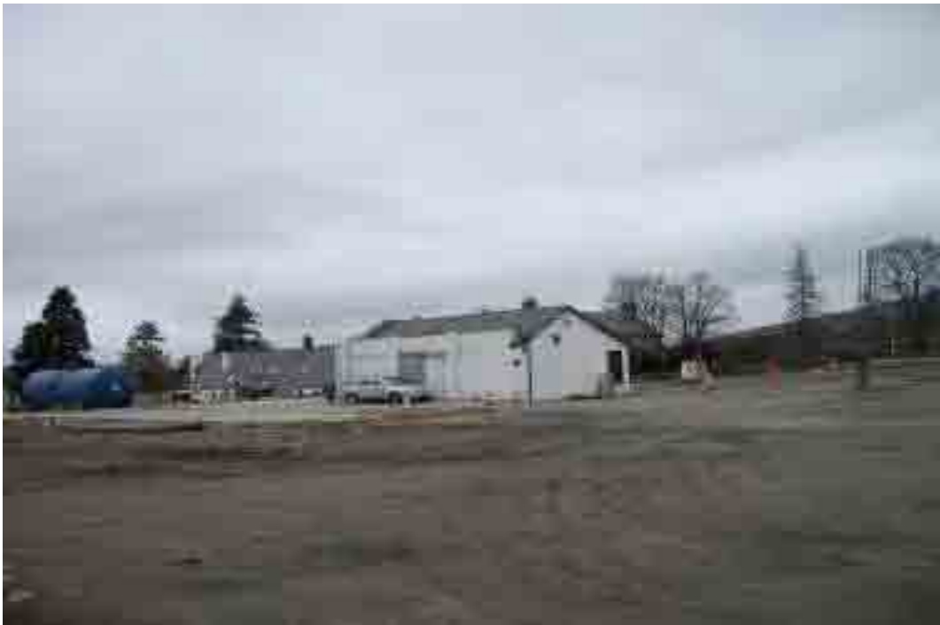
Eastern section, showing J4 hardstanding and adjacent garage
