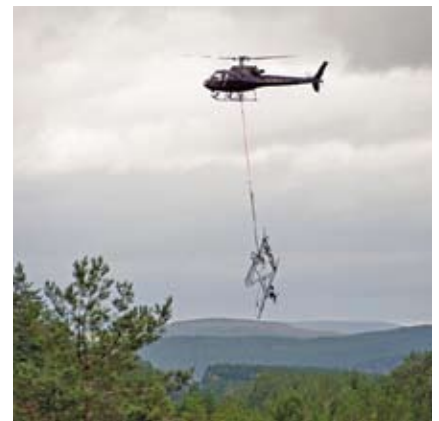
Redundant pylons being removed from Dell Woods, Nethybridge © David Gowans
