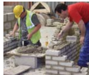
Laying the foundations for the future © The Highland Council
