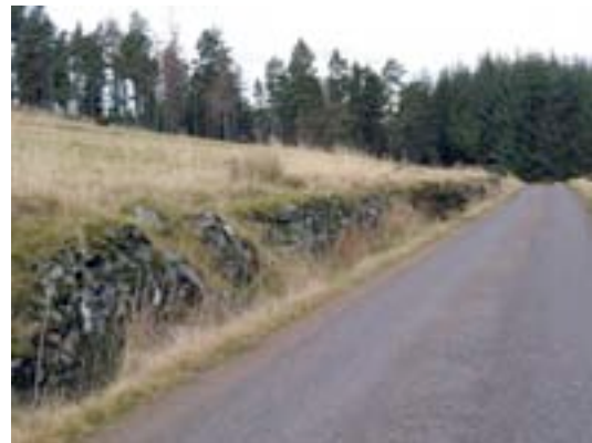
Stone retaining walls along the 'upside' of the narrow roads
