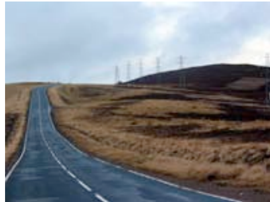
The road sits on the edge of the valley, sometimes on an exposed ridge
