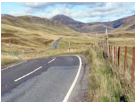
The road hugs the landform, following its ridges and dips, here the verge defined by a metal fence
