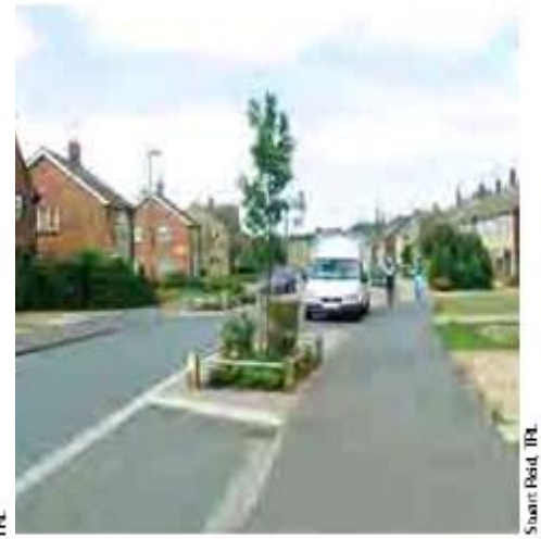
Figure G7.4 Kerb build-out defines parking area and provides room for planting clear of the footway.
