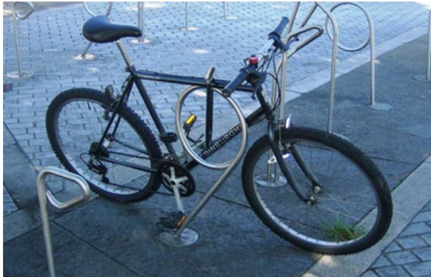
Figure G5.4 A contemporary design for cycle parking - note that this arrangement is not so convenient for locking both wheels to the stand (WSP, Scottish Parliament).
