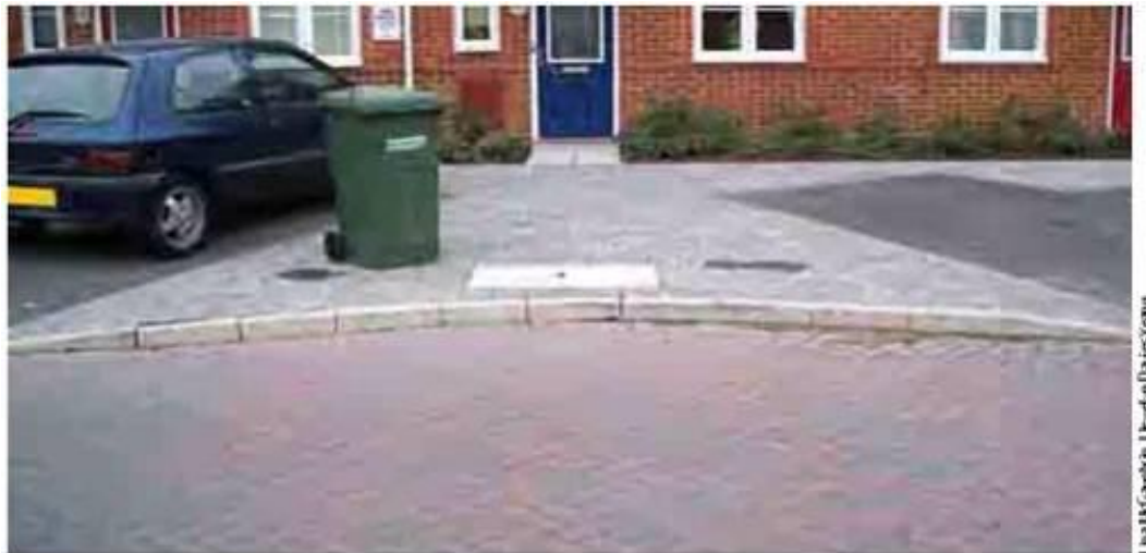
Figure G5.11 Street detailing and pedestrian provision dominated by car-parking considerations.
