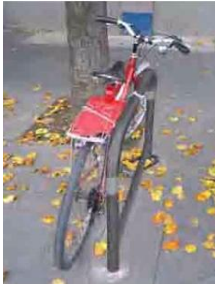
Figure G5.3 Sheffield stands are simple and effective. The design allows the bicycle frame and wheels to be easily locked to the stand. Note the tapping rail near ground level and the reflective bands on the uprights.
