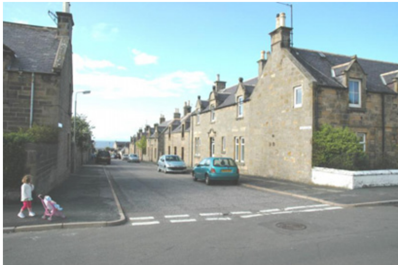
Figure G4.10 Quadrant kerbstones used instead of large radii at junctions reduce the dominance of the carriageway. This is reinforced by the placement and form of the adjacent buildings. However, note the lack of dropped kerbs and tactile paving (WSP, Hopeman).
