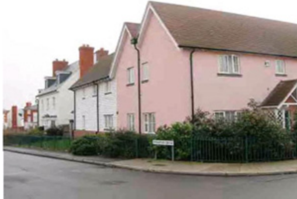
Figure G1.11 Active frontage to all streets and to neighbouring open space should be an aim in all developments. Blank walls can be avoided, even on the return at junctions, with specially designed house types.
