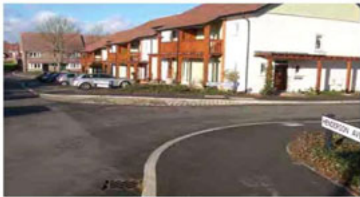
Figure G4.24 The overrun area at this junction is hazardous for pedestrians and/or requires them to divert from their desire line. Notice also the unsightly placing of inspection covers. The layout is particularly hazardous for blind and partially-sighted pedestrians.
