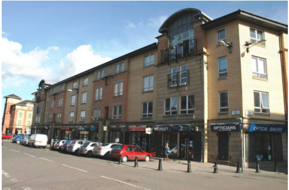
Figure G5.10 On-street parking in Crown Street, Glasgow (WSP).
