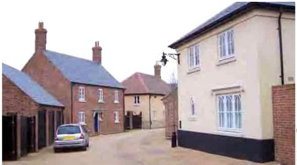
Figure G8.3 Street light mounted on a building.
