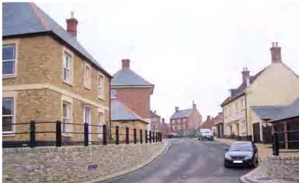
Figure G3.11 In some instances it may be possible to keep footways level when the carriageway is on a gradient, although this example deflects pedestrians wanting to cross the side road significantly from their desire lines.
