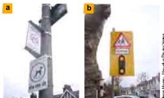
Figure G7.1 (a) Sign clutter in residential areas; (b) the yellow backing board adds clutter and its use with the flashing amber lights is counter-productive. In addition, the sign post should not protrude above the sign.
