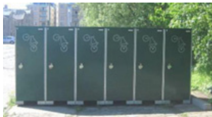
Figure G5.1 Secure cycle storage (WSP, Leith).
