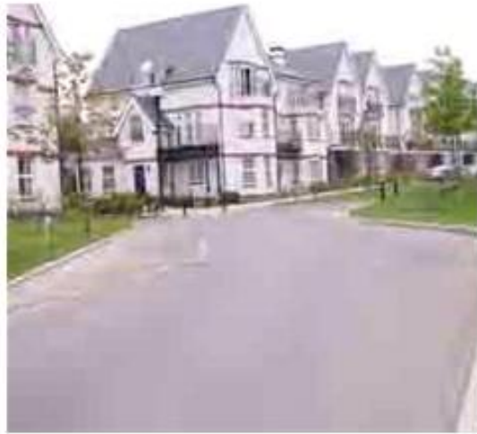
Figure G7.3 Street with no centre lining.
