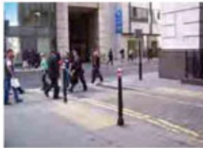
Figure G3.4 Raised crossover, but located away from the desire line for pedestrians and therefore ignored - the crossover should be nearer the junction with, in this case, a steeper ramp for vehicles entering the side street.
