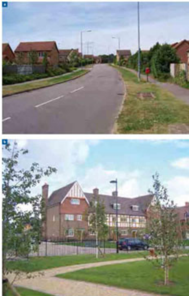
Figure G1.13 (a) Existing development in Upton turns its back on the street; while (b) a later development has a strong presence on the street. The latter was delivered using a collaborative workshop design process and a design code.
