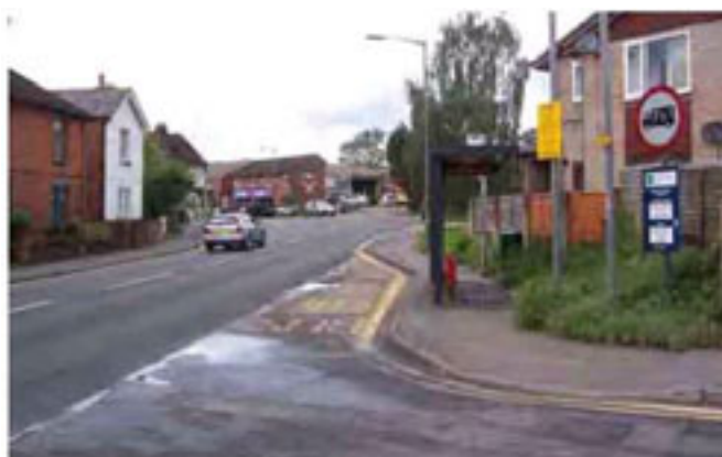
Figure G3.17 The bus lay-by facilitates the free movement of other vehicles but it is inconvenient for pedestrians.
