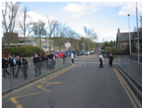
Figure G8.2 Guard railing blocking pedestrian desire line - note some pedestrians in the photograph have walked around it (Ellon, WSP).
