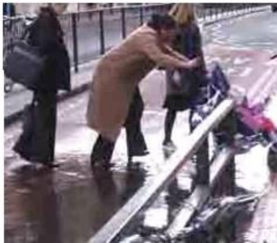
Figure G3.13 Poor drainage at a pedestrian crossing place causes discomfort and inconvenience.
