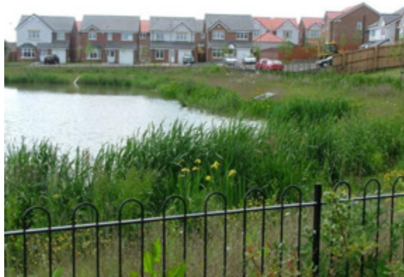
Figure G6.5 Sustainable drainage systems can form an integral and attractive part of the street (WSP).
