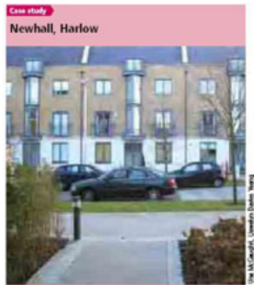
Figure G4.2 On street parking and shallow gradient junction table suitable for accommodating buses.
