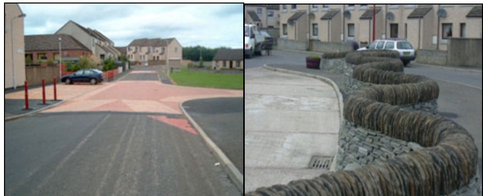
Fig G4.8 (a) Raised speed table Lord Thurso Court, helping to reduce vehicle speeds and facilitate pedestrian movement (b) wavy wall created using local Caithness Stone aiding the sense of context and place identity (Scottish Executive 7 ).
