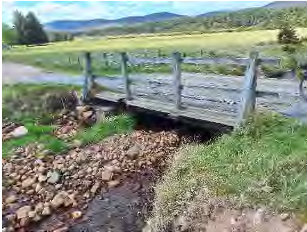
IMAGE 1 - EXISTING VEHICULAR BRIDGE TO BE DEMOLISHED AND REMOVED
