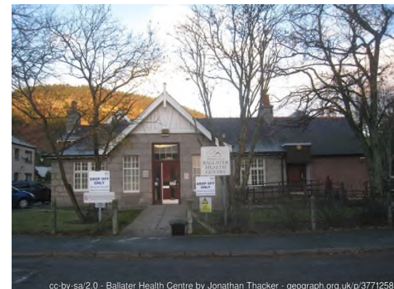
Figure 1 – NHS Grampian Ballater health centre
