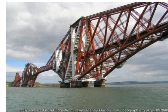
Figure 3 – perhaps the most infamous repair project in Scotland, painting the B listed Forth rail bridge (now done on a ~20 yearly basis)
