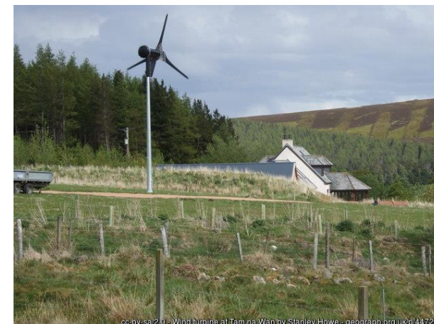
Figure 4 – free standing small scale turbine
