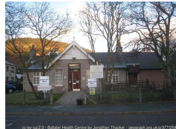
Figure 1 – NHS Grampian Ballater health centre
