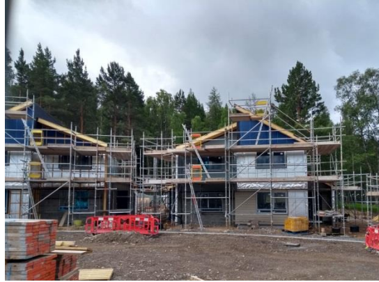
Figure 2 – affordable housing under construction at Inverdrurie, near Aviemore
