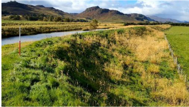
Figure 3.60. Fencing positioned along the dry side (furthest from the channel) of embankments and river corridors to mitigate against trampling by livestock.
