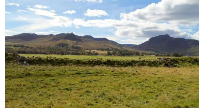
Figure 3.62. Lowering of the embankment crest to form a spillway (formalised embankment breach) at Breakachy Farm (OS NGR NN 64187 93793).
