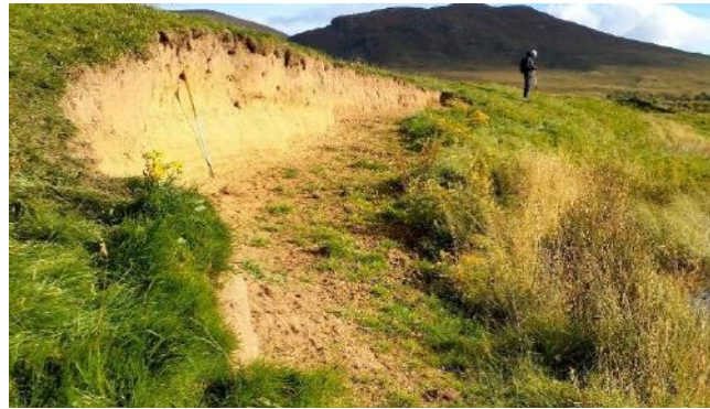
Figure 3.2 Moderate-severity riverbank erosion.
