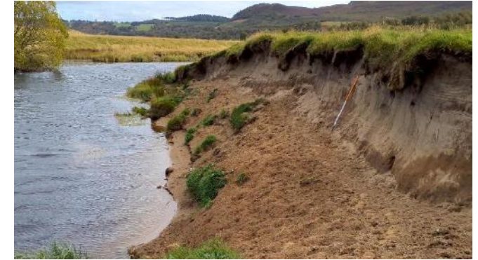
Figure 3.3. High-severity riverbank erosion.
