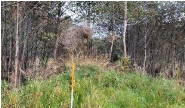
Figure 3.10 Young tree growth and regeneration across the crest and face of an embankment.
