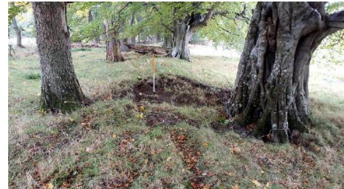
Figure 3.65 Example of mature trees growing on the embankment and erosion caused by sheltering livestock.
