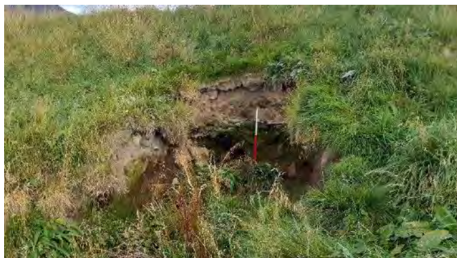
Figure 3.63 Culvert through the embankment with erosion around the inlet at Drumgask Farm (OS NGR NN 61927 94037).
