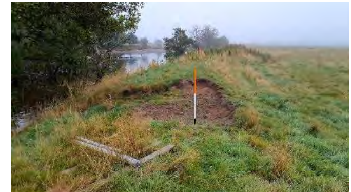
Figure 3.6 High risk of embankment breach. Embankment positioned along the top of the riverbank. Bare ground and slumping evident across over half of the embankment crest width.
