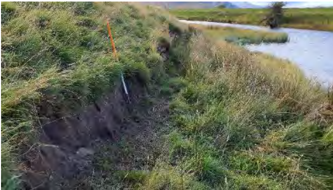
Figure 3.1. Low-severity riverbank erosion.
