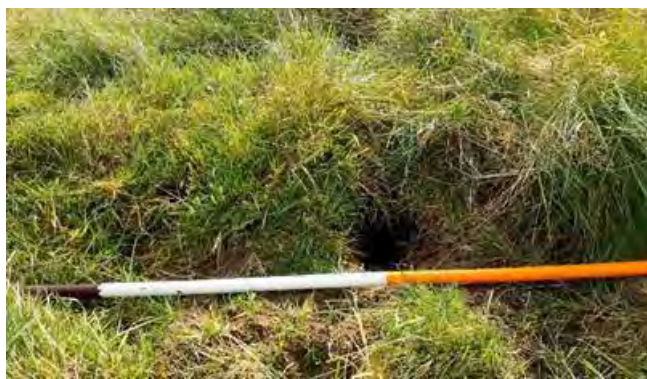
Figure 3.11 Burrow within the crest of an embankment. Mole hills and burrows were occasionally noted in Areas 1 and 2, but their position and density were insufficient to cause concern at the time of survey.
