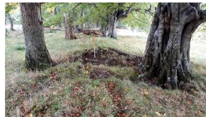
Figure 3.65 Example of mature trees growing on the embankment and erosion caused by sheltering livestock.
